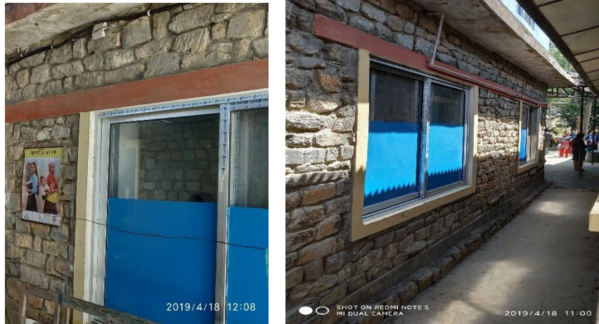
Figure 11: Replacement of wooden frames to windows
