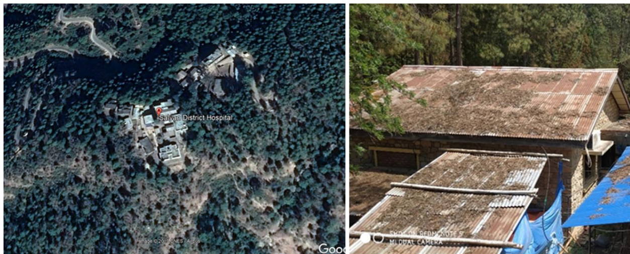
Figure 5: Salyan Hospital surrounded by forest (left) and dry pine leaves on building roofs (right)
