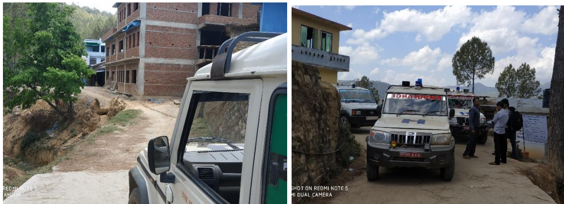
Figure 10: Access road to Emergency block
